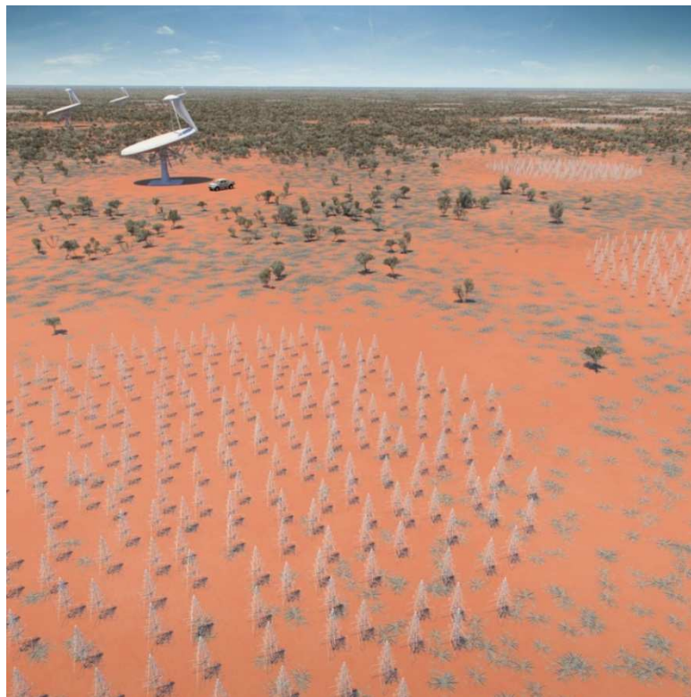
Artists impression of the low-frequency aperture array of the SKA to be based in the Australian Murchison region. Image courtesy of the SKA Telescope Organisation
