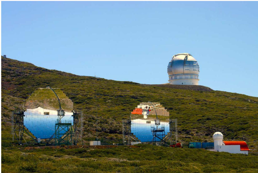
The two 17m diameter gamma-ray telescopes of the MAGIC Observatory on the island of La Palma with the Gran Telescopio Canarias (GTC) in the background. Photo courtesy of Robert Wagner, Stockholm University.
